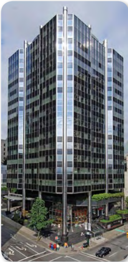
Above: Grant Thornton Place in Vancouver, Go Green certified
